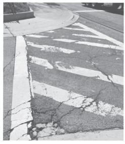
roadways, we have no idea as to the condition of the foundation beneath the asphalt topping and will only know that after the milling process.
